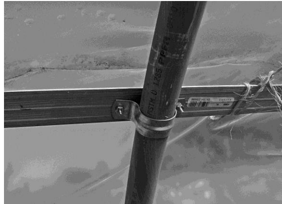
Purlin along hoop- simple pipe clamp and molding
