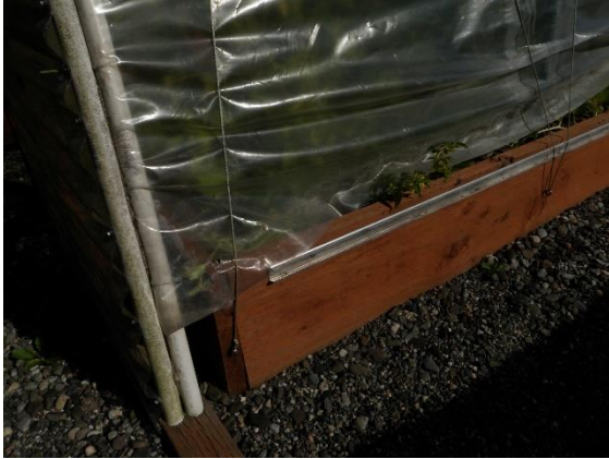
Wind stability additions: Channel lock along base
